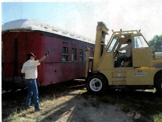
Above left – Jeff Gardner of Nielson-Skanska Construction Co. supervises the initial lift of the coach from the old foundation. Above right – the coach is moved onto the street by a pair of heavy-duty forklifts for loading onto the truck.
