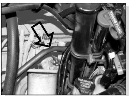
Damaged discharge line shown.
