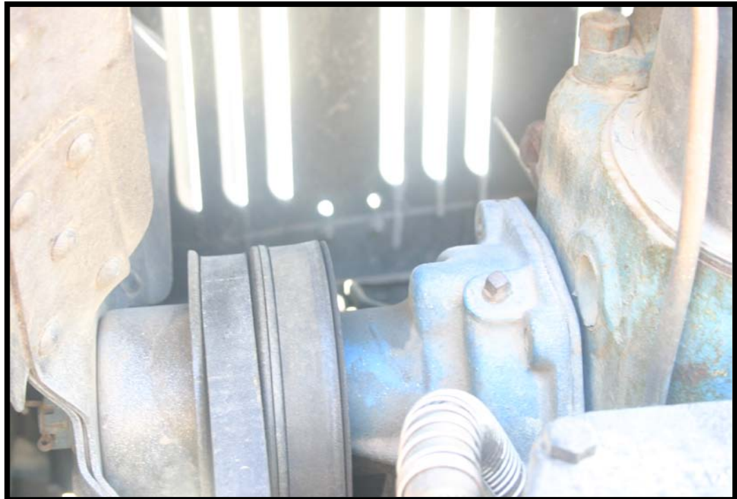
Fan, water pump, pulley
