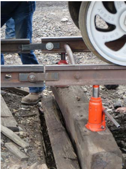
Ties and Bottle Jacks used to support and stabilize the rails.
